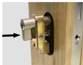
3. Remove the thumb turn from the cylinder by pushing in the release pin on the thumb turn or by using an allen key where appropriate. Next, install the cylinder into the lock in the door leaf from the external side. Install the cylinder in the normal manner aligning the cylinder retention screw through the lock face-plate.
