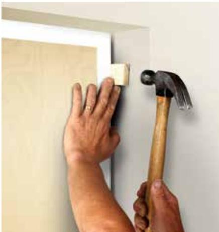
3. After ensuring the hinge jamb is square and plumb by re-adjusting the wedges if necessary, fix the hinge jamb in four positions (as shown).
