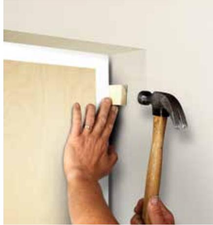
2. Hold the frame in place using wedges, ensuring the frame is square. A large (5ft/1.5m recommended) spirit level should be used to ensure that all jambs are square and plumb.
