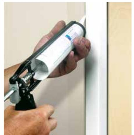
6. The frame to wall gap must be filled with mineral rock fibre tightly packed to a depth of the frame leaving an allowance for a 10mm capping, to both faces, with BS467-20 tested fire rated mastic. Alternative options can be found in BS 8214.
