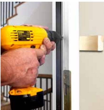
4. Close the door and position the closing jamb so that it makes full and uniform contact with the frame seal. Then fix (as step 3).
