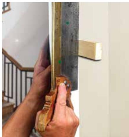
5. Cut off the wedges to align with the edge of the frame.
